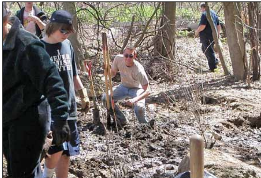
Planting native trees and shrubs in the riparian zone helped restore and stabilize the stream bank.
